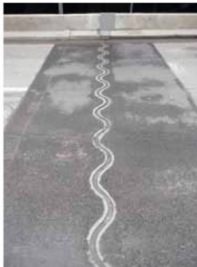
12 Wave shaped single seal expansion joint © Maurer Söhne GmbH & Co. KG
