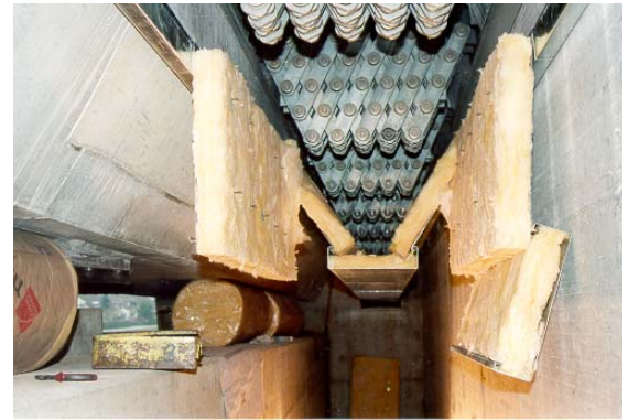
So called „Scissor Control“ of a joint, to be covered by a partially mounted folding system.
