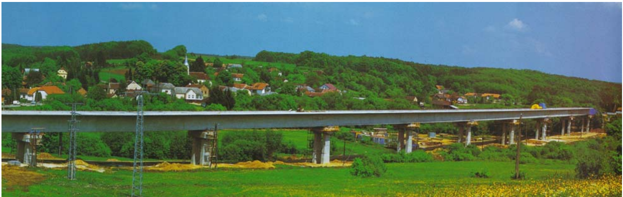
Railway Bridge Zalalövö-Bajánsenye/Hungary (1999 – 2000), 82 pot bearings, vertical load up to 12,000 kN
