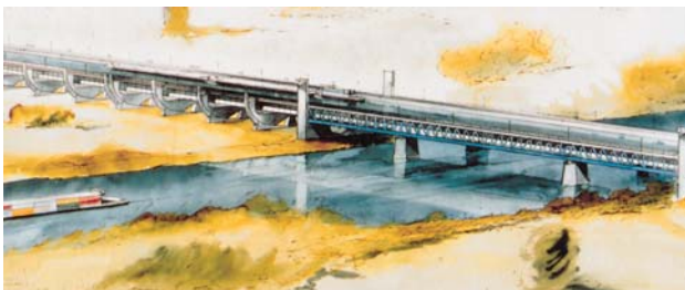
Canal Bridge Magdeburg, Trough Bridge over the river Elbe, 2000 – 2001 4 spherical bearings for vertical loads up to 131,000 kN (with spherical- \varnothing 2,200mm) 4 spherical bearings for vertical loads up to 18,000 kN
