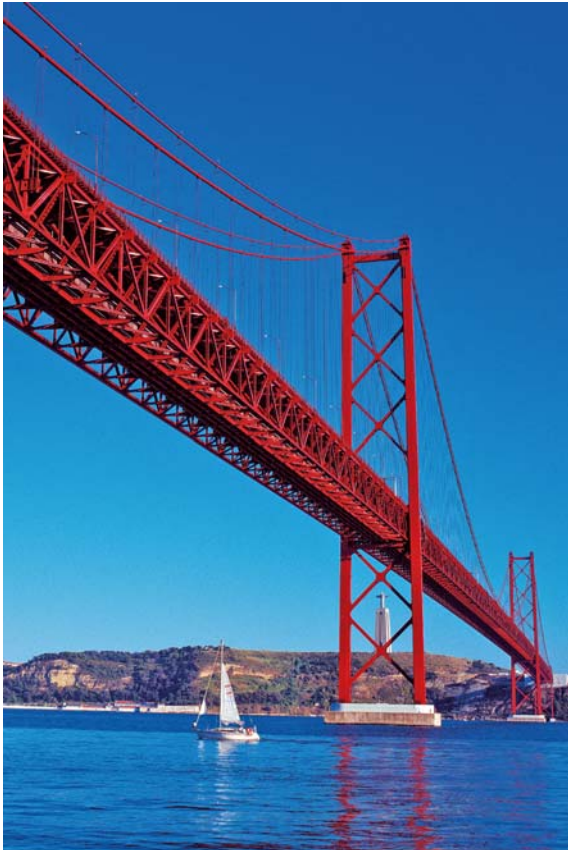
The bridge „Ponte 25 de Abril“ links Lisbon with Almada. At the 2 abutments and at the cable bearer piers, roller bearings were replaced by MSM spherical bearings
