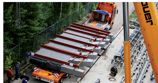
Transportation of the world's biggest expansion joints with noise protection elements.
