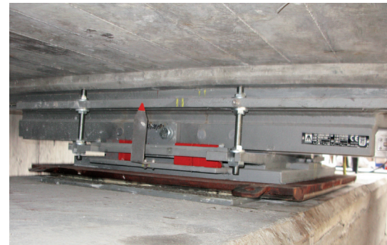
Fixed MSM Spherical Bearing at the abutment (axis 100) prior to lateral shifting.
