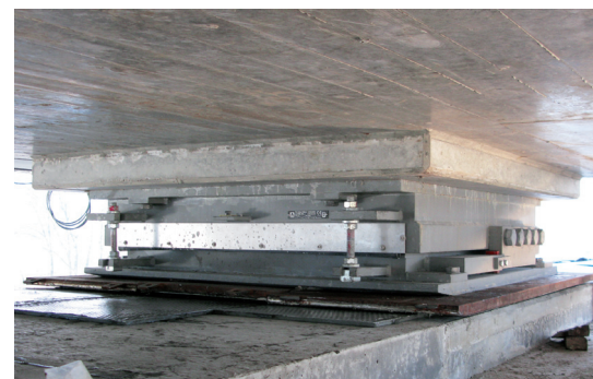
End position of the MSM Spherical Bearing after lateral shifting. The bearing is still fixed on the shifting sledge.
