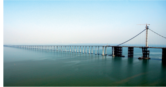
The Qingdao-Haiwan-Bridge at the area of the suspension bridge, where expansion joints of up to 1,120 mm movement capacity are installed.
