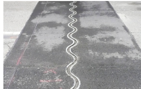
World wide first installation of the wave shaped expansion joint at Donnersberger Bridge Munich. Photo: Maurer Söhne
