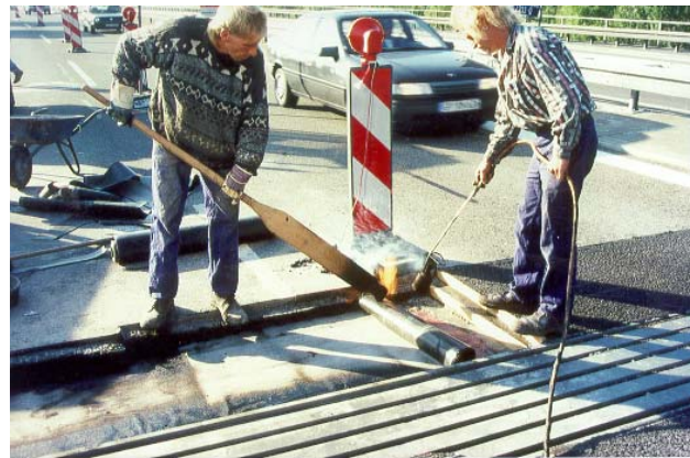
The watersealing is applied in hot state
