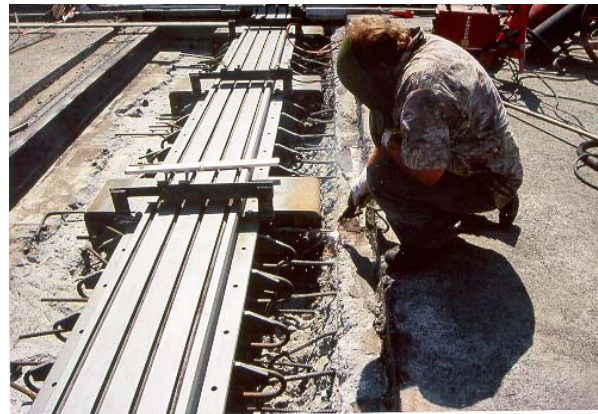
Tack welding the reinforcement in the recess with the anchor loops of the joint.
