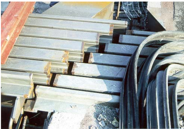
Levelling and adjusting the new modular joints in the recess.
