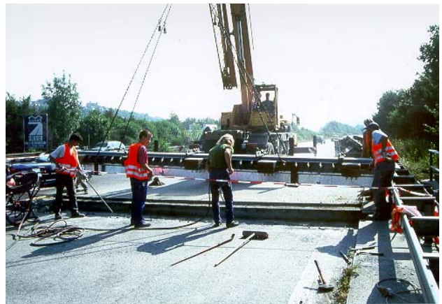
Lifting the new modular joint into the structural recess.
