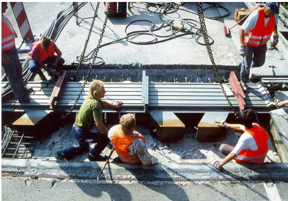
Levelling and adjusting the new modular joints in the recess.
