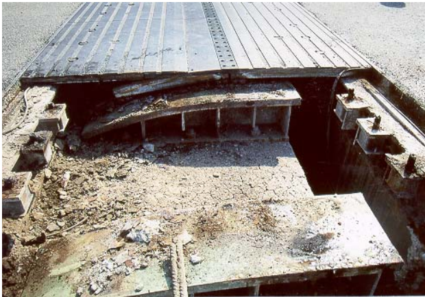
Removing the existing roller shutter joint lane by lane
