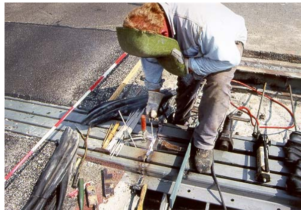
Tack welding the reinforcement in the recess with the anchor loops of the joint.
